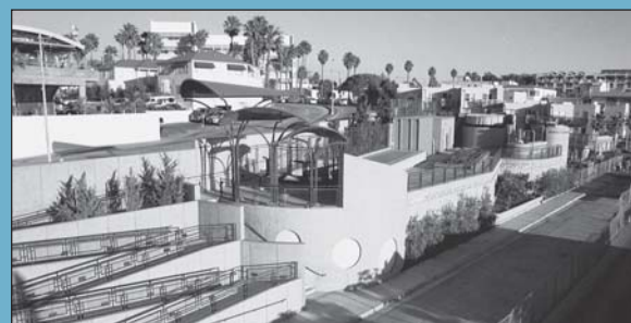
The Santa Monica Urban Runoff Facility (SMURRF). This innovative park-like facility helps the city meet Clean Water standards for the Bay and could serve as a model for future CEQA water quality mitigation measures.
