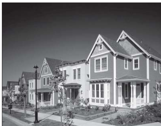
Now that contamination issues have been addressed, construction has begun on the Hercules Transit Village. Each home meets design guidelines to blend-in with Hercules' historic buildings.
