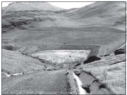
CEQA review led to important environmental mitigations such as this sedimentation basin which collects stormwater run-off and prevents sediment from leaving the site.
